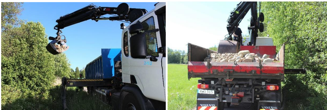
Figure 91. Two crane trucks were used to deliver the stones. Photo Mikael Lindén
