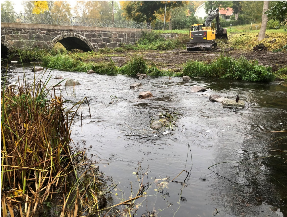
Figure 79. Stretch 1a, Skebobruk, during implementation. A multichannel stretch is recreated. Photo credit: Patrik Bergquist.
